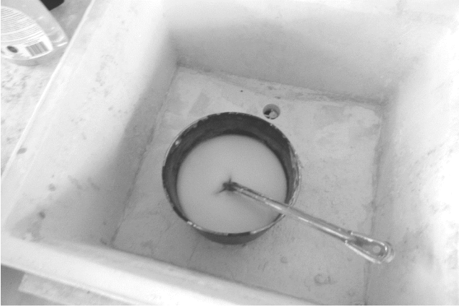
36 The dry plaster is mixed with water and stirred.
