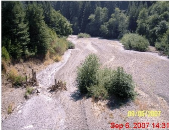
A dry South Fork, looking upstream from the South Fork bridge at Twin Bridges.
